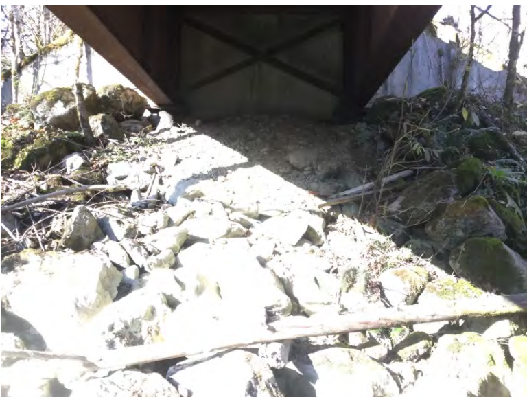
Right Bank Abutment when facing downstream
