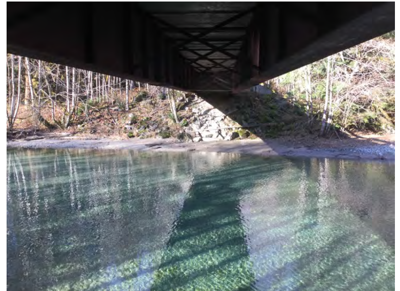
Right Bank Abutment when facing downstream
