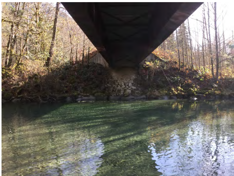
Left Bank Abutment when facing downstream
